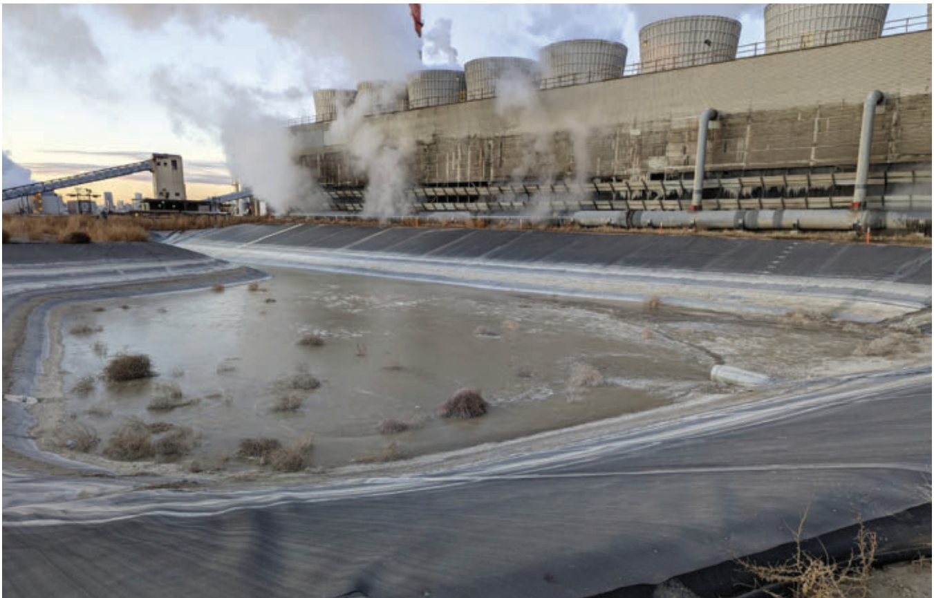
Figure 5: Equalization pond with several hundred thousand pounds of sludge filling the bottom three feet of the pond.
